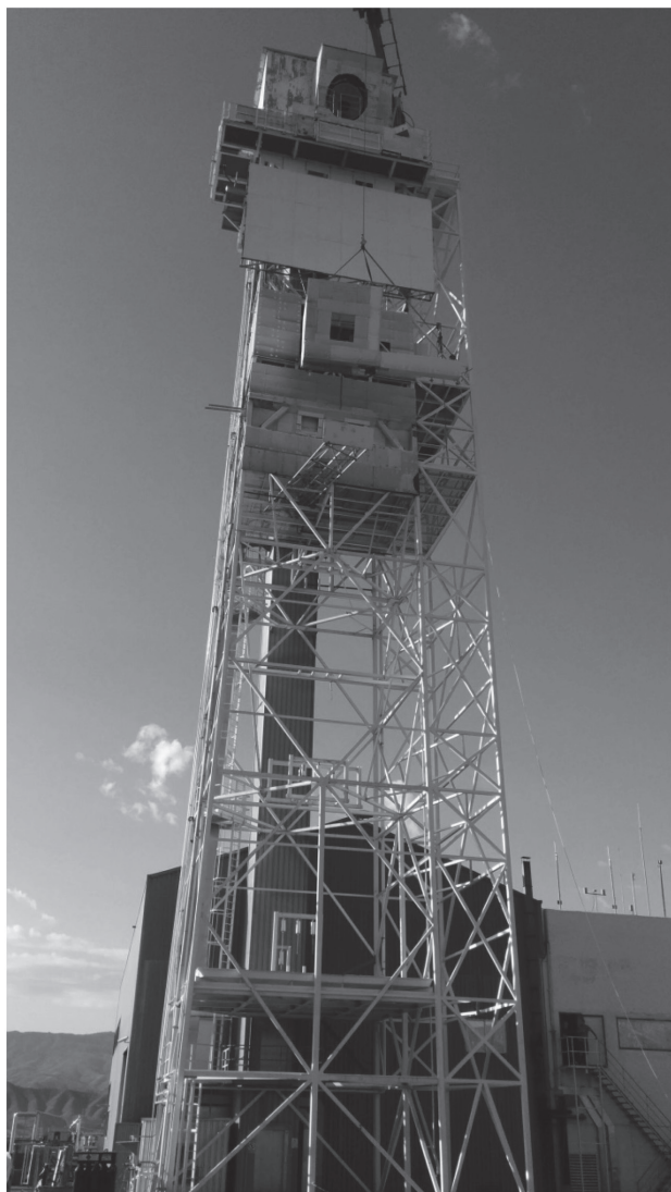
Fig. 1 SSPS-CRS tower at CIEMAT-PSA, Almería. Solar reactors from SYNPET, SOLH2 and HYDROSOL are installed in different height platforms from top to bottom (courtesy: Abengoa Hidrógeno)
